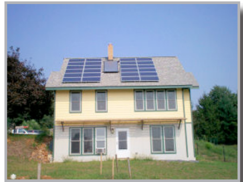
Residential solar panel installation
